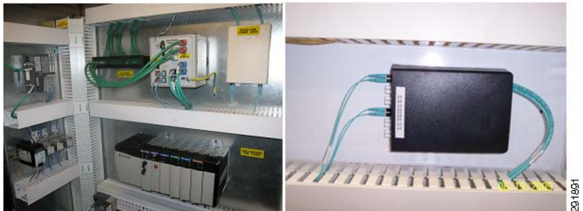
Figure 9 Sample Control Panel Fiber Optic Deployment
