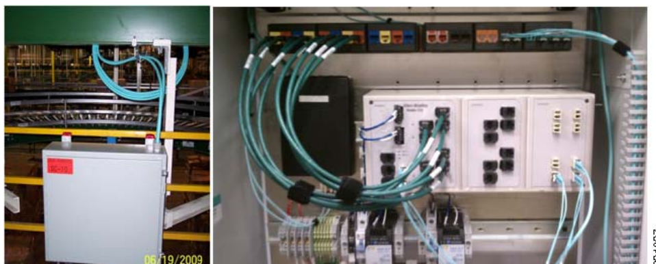
Figure 11 Sample Network Zone Fiber Optic Deployment
