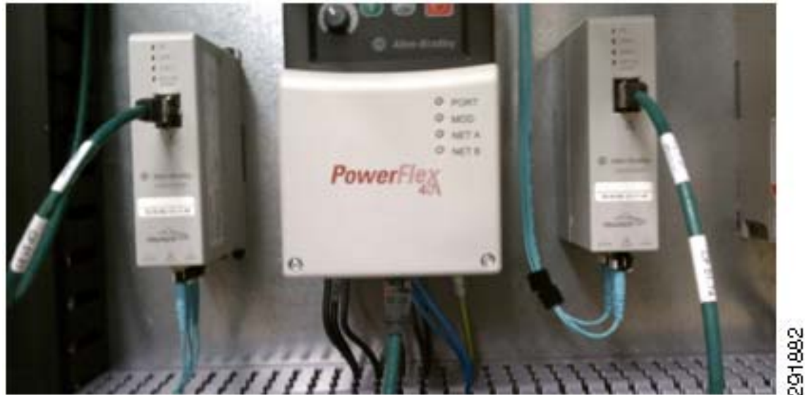
Figure 5 Sample Device-Level Fiber Optic Deployment
